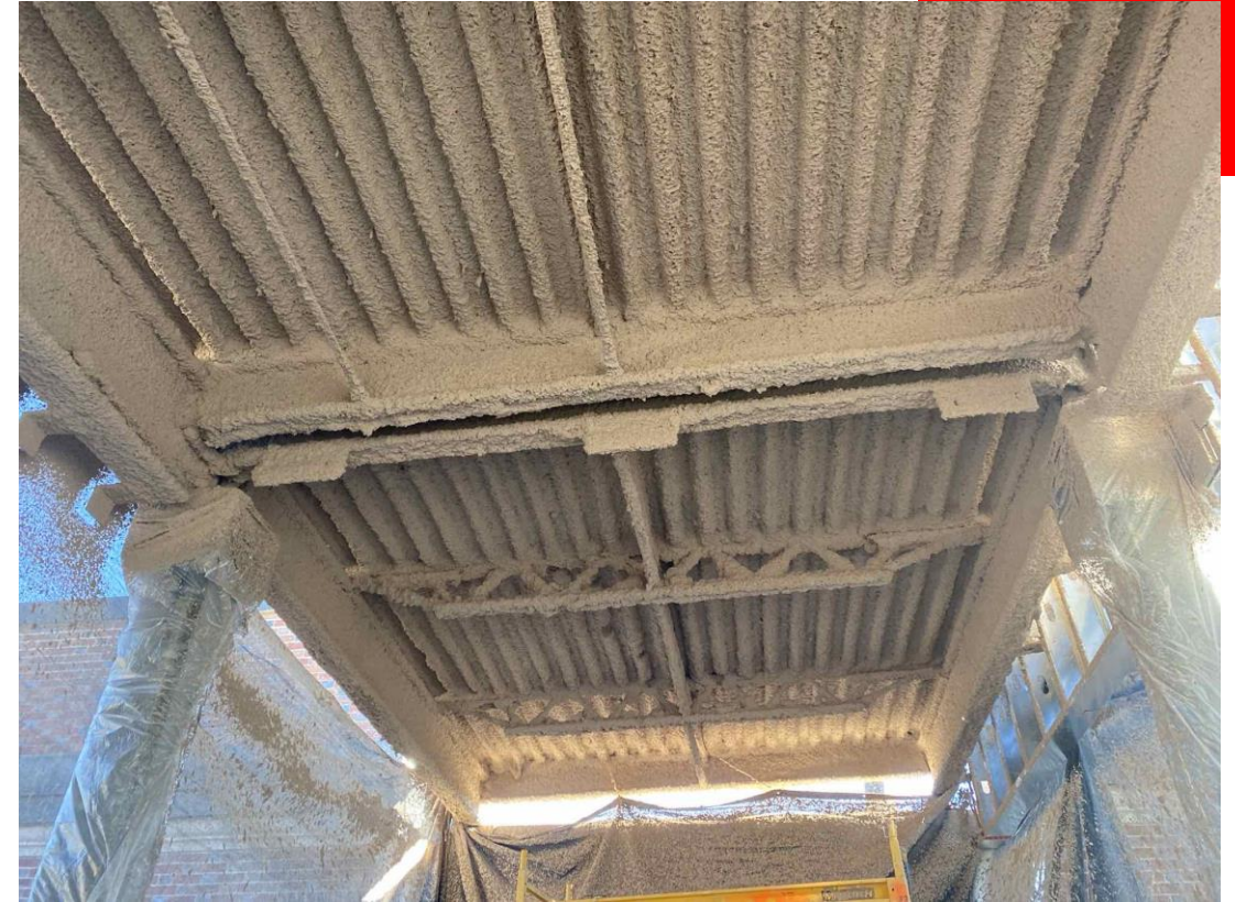
Fire Proofing Completed at New Addition Bridge
