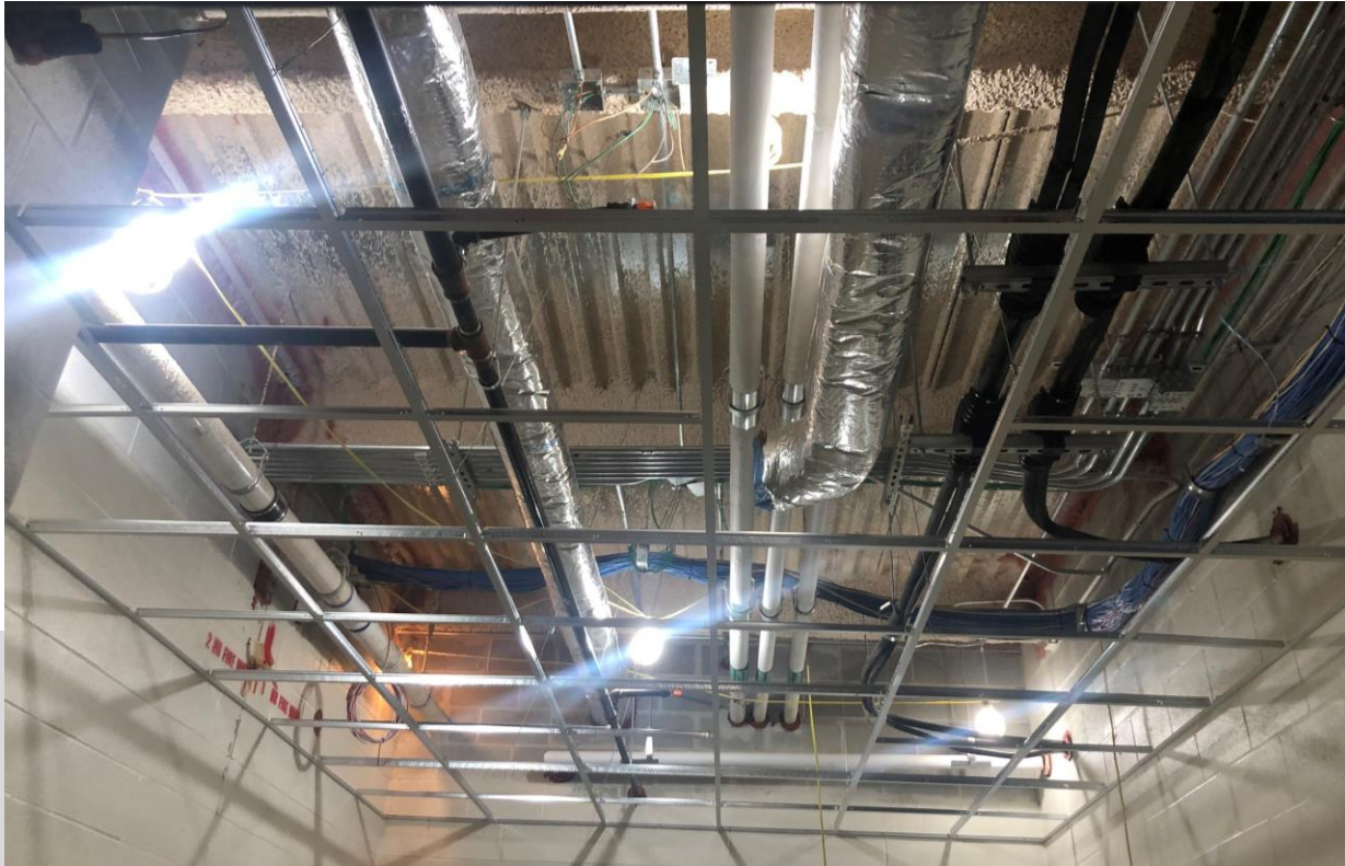
ACT Ceiling Grid Installed First Floor of New Addition
