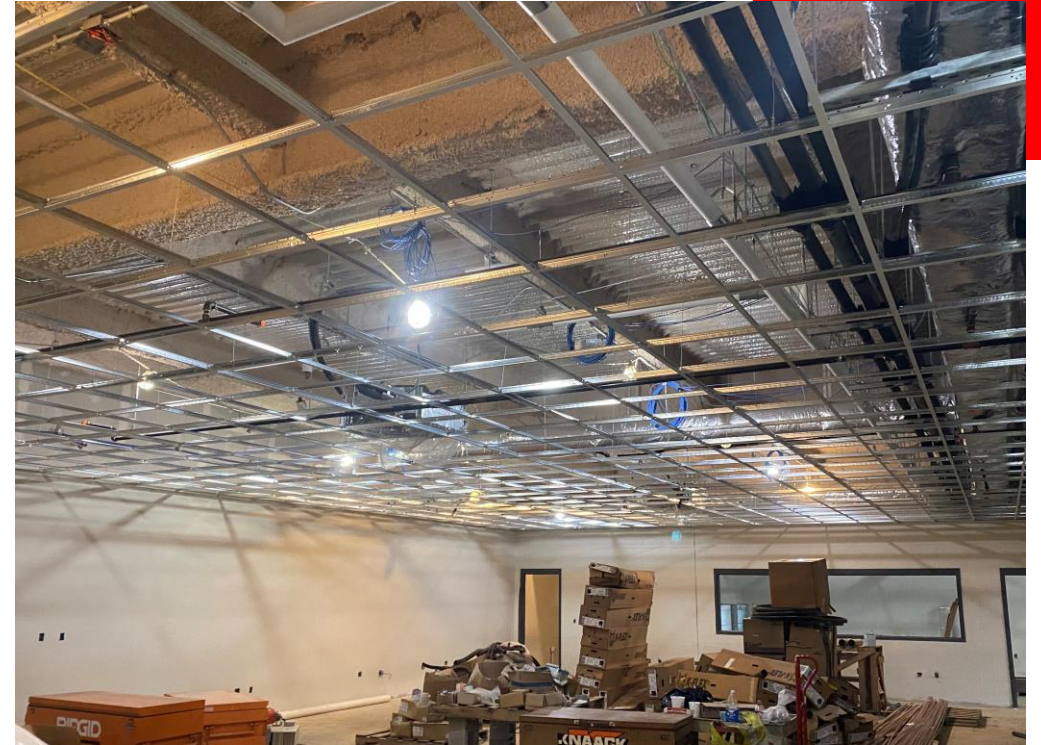
ACT Ceiling Grid Installed First Floor of New Addition
